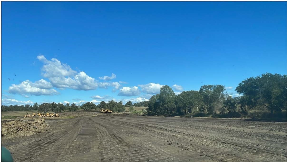
Figure 2: View of the Stripped Surface
