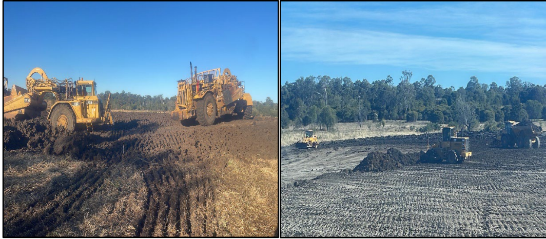
Figure 3: View of the Filling Operations
