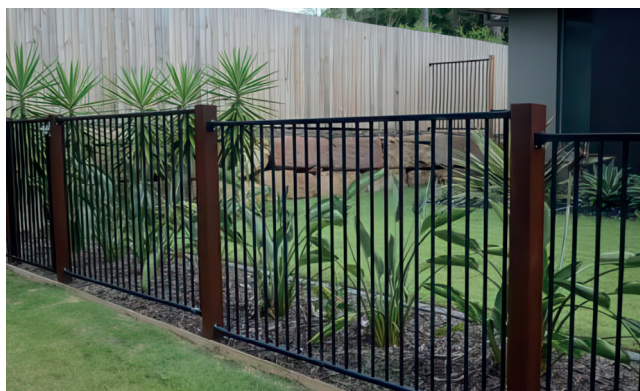
Example of Pool Fencing
