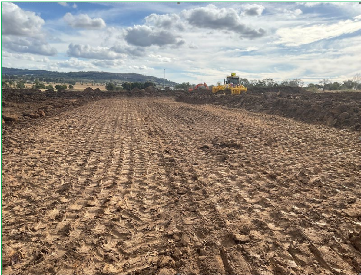
Figure 4: View of Filling Operations
