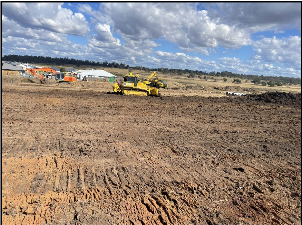
Figure 3: View of the Stripped Surface on Stage 6B1 and 6B2
