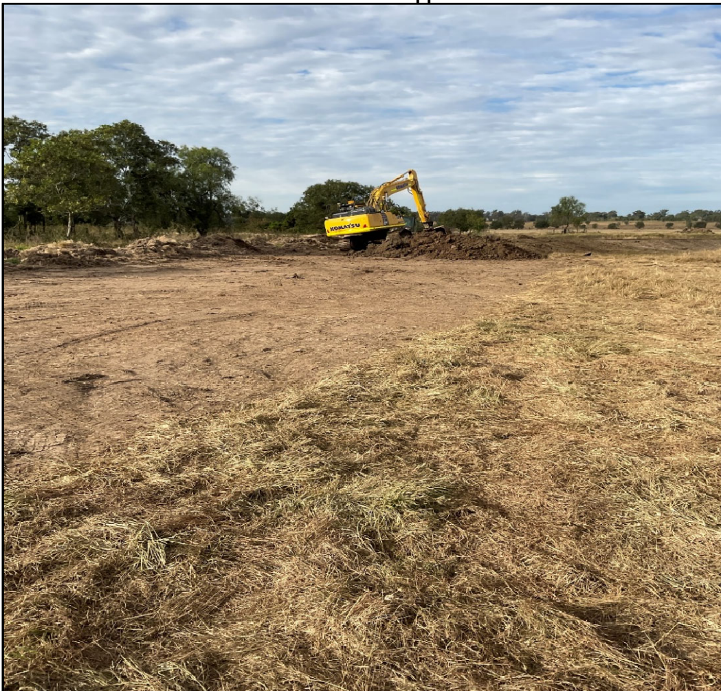
Picture 1: View of the Stripped Surface
