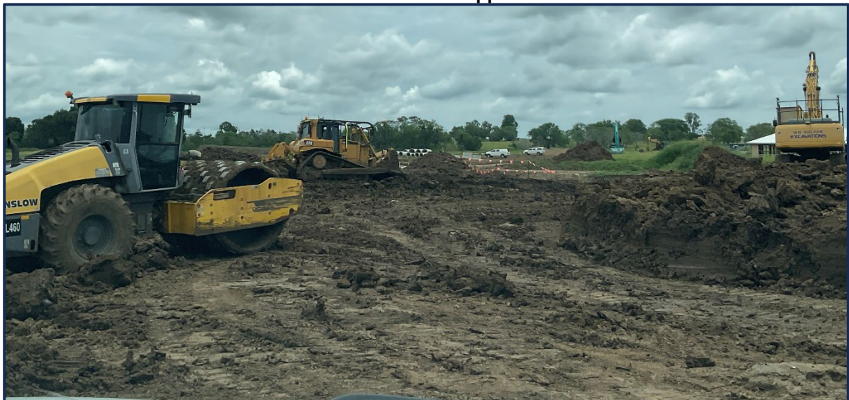
Picture 1: View of the Stripped Surface
