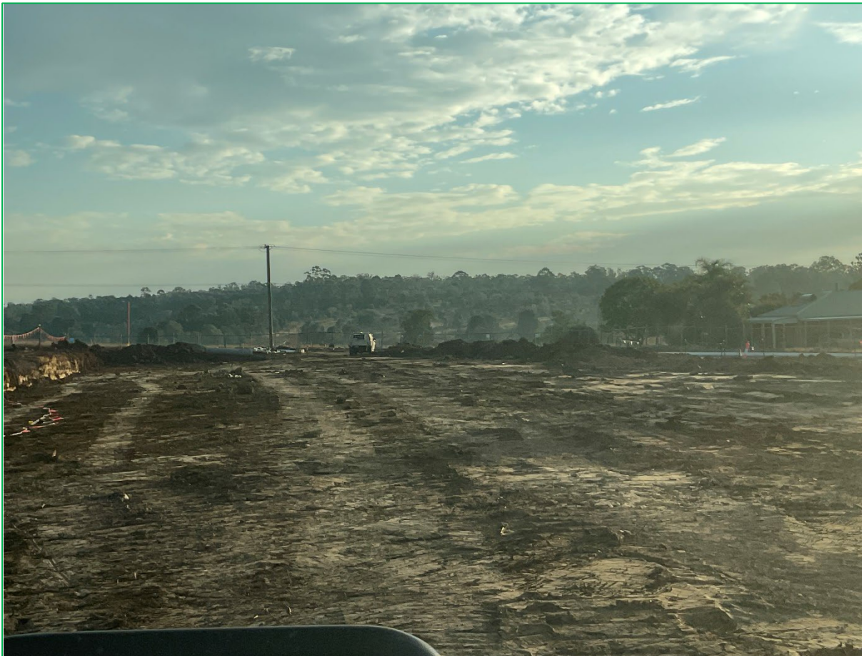
Picture 2: View of the Stripped Surface on Stage 1 Gibbs
