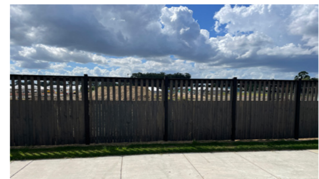
Example of secondary frontage or park facing fencing with 50% transparency above 1200mm
