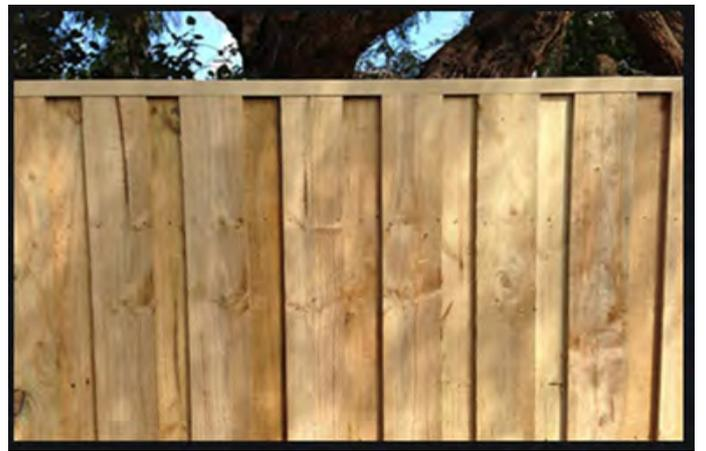
*Example lapped and capped timber fencing*
