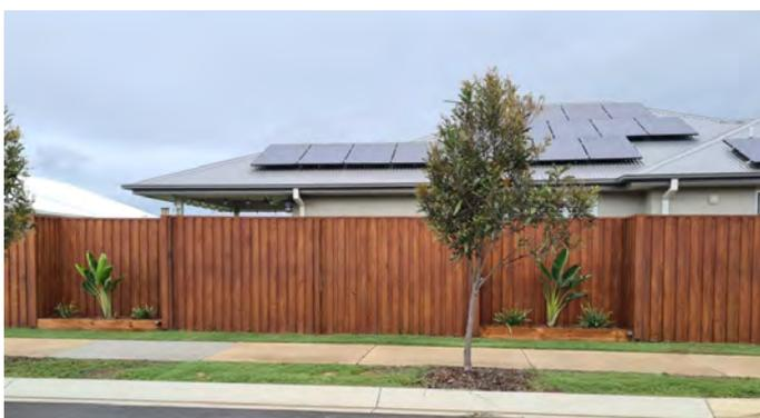
*Example lapped and capped side fencing*
